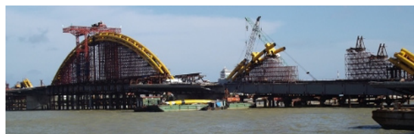
Figure 15. Construction of steel arch [foto by Ehrin Macksey/Noi Pictures].
