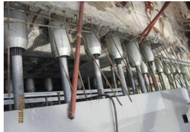
Figure 12. Prestress cable between steel and concrete section.
