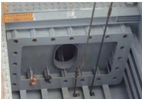
Figure 9. Prepare steel girder to transport.
