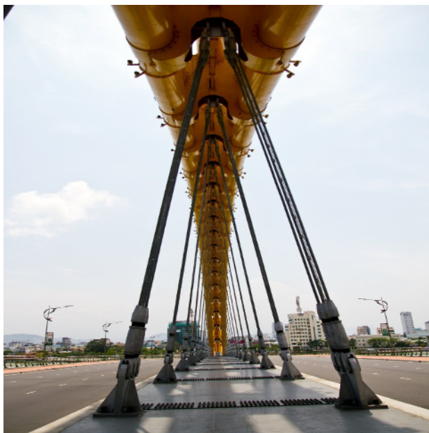
Figure 13. Steel hangers.
