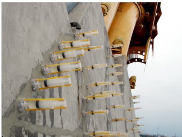
Figure 17. Injection epoxy glue to fill the cracks.
