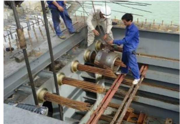
Figure 11. Cable tension in joints between sections.
