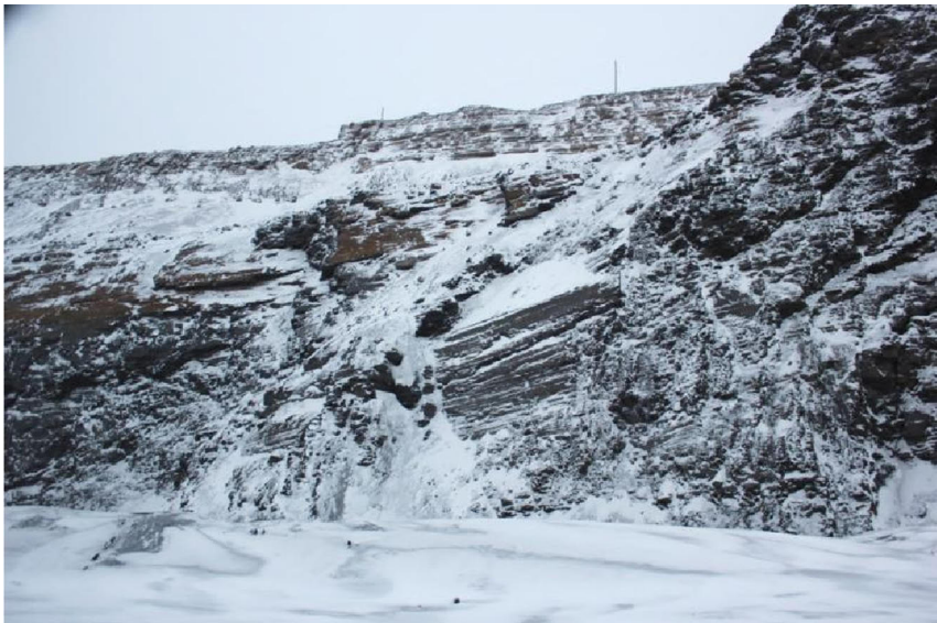
Fig 4. The site of the first bench in the collapse area.
