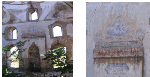
Fig. 3. Photographs before and after restoration of the Timurtaş(Demirtaş) Mosque (2007).
