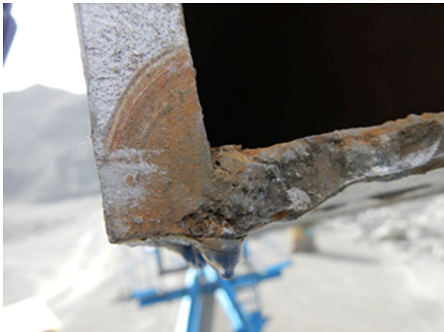
Fig. 3. Fracture of a mining shovel boom metallic structure.
