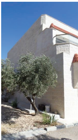
Figure6. Western elevation, Al-Kamaliya house Reference: Researchers
