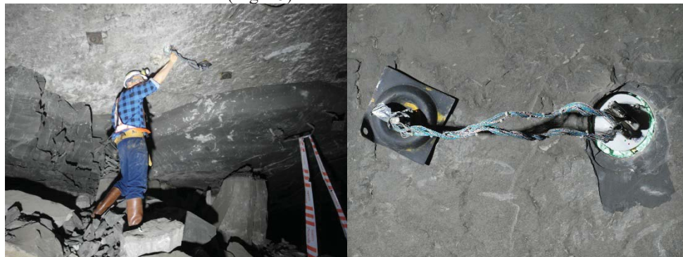
Fig. 15. Installation of instrumented rock bolt.
