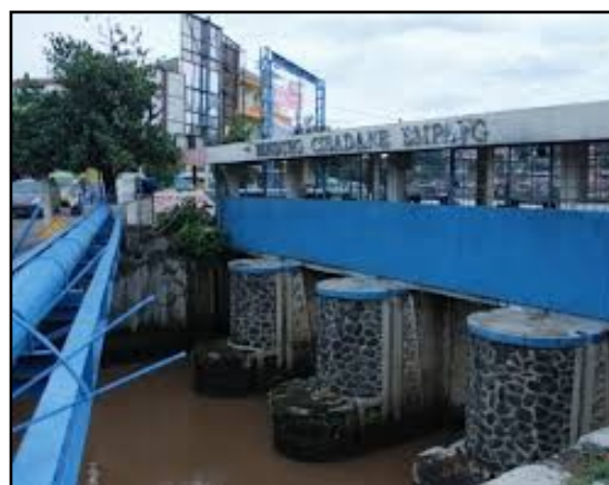
Fig. 3. Water gate for irrigation system in Empang, Bogor
