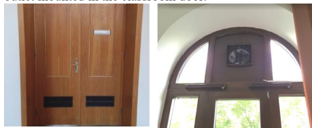
Fig. 2. Photos with the window fan + hygro-adjustable grids and the extraction outlets in the door
