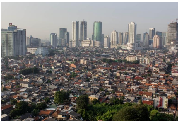
Fig. 10. Newer high-rise buildings juxtaposed with the traditional, low-rise urban context of Jakarta. (Source: CC BY-SA Magdalinski).
