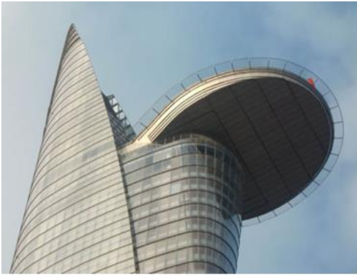
Fig. 10. The helipad of the tower. [ Source: DESIGN.VN ]
