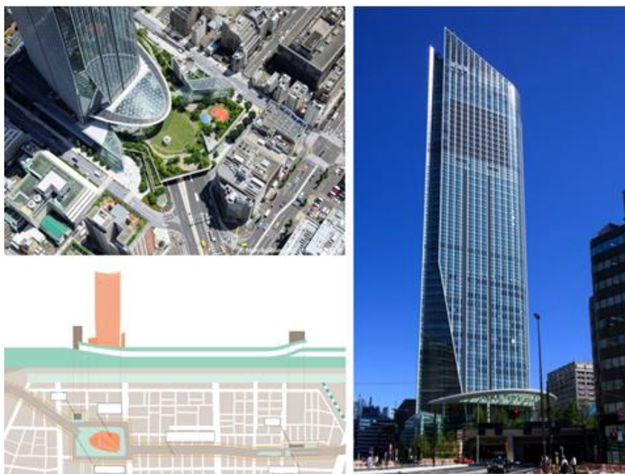
Fig. 2. «Toranomom Hills», Japan, Tokyo, 2014, 258 m, 52 floors, designed by Nihon Sekkei [12].
