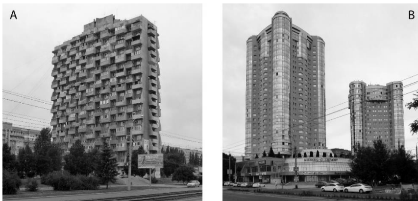
Fig. 1. The first high-rise residential buildings in the city of Samara.
