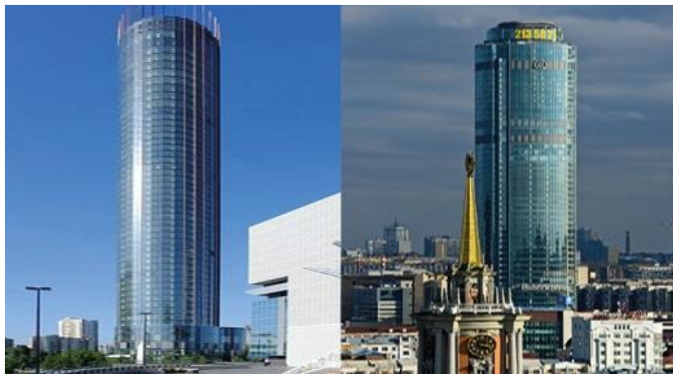
Fig. 2. Two highest skyscrapers of Yekaterinburg: the Iset Tower residential complex, overall view (left), Vysotsky business center, overall view (right) [13, 8]
