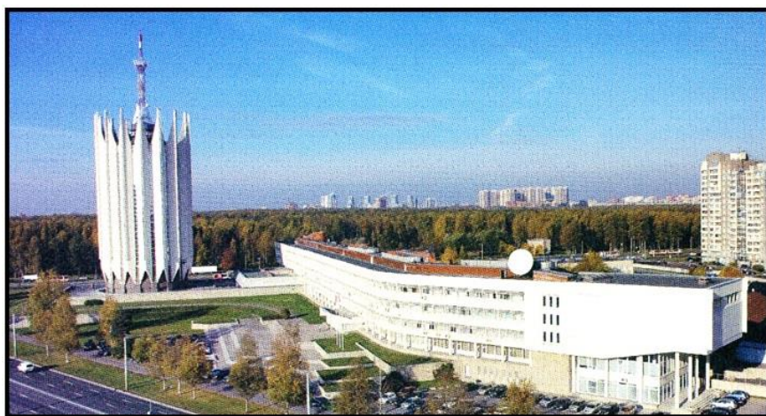
Figure 10. High-rise complex of the Central Research and Development Institute of Robotics and Engineering Cybernetics (1973–1986)
