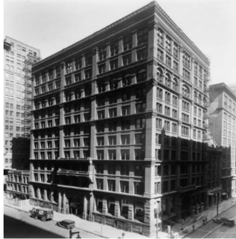
Fig. 1. Home Insurance Building – Chicago [1]
