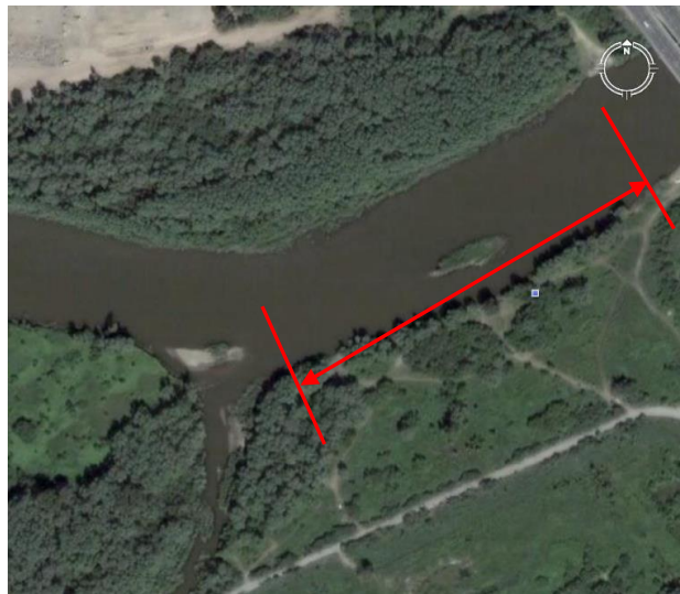
Fig 2. Space shot of the channel section
