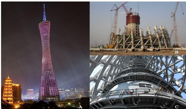
Fig. 1. The "Canton Tower" TV Tower with the height of 600 m (Guangzhou). a - the general view of the tower; b - course of construction, c - shell of tube confined concrete elements.
