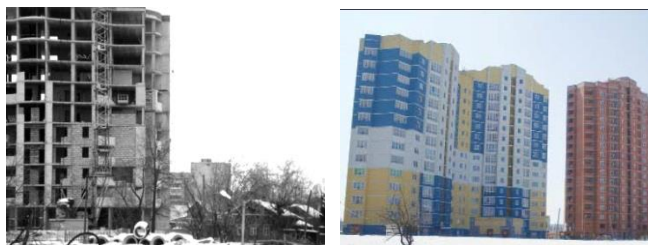
Fig. 4. Construction of a multistory building.
