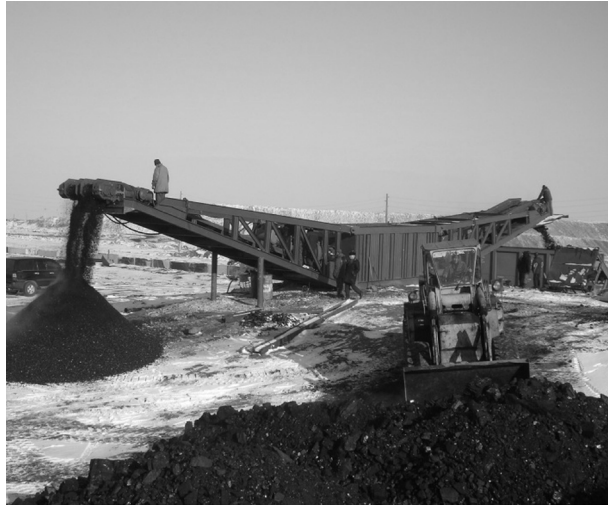
Fig. 2. Design of a DSKA complex, capacity 750 t/h, Karazhyra open pit mine, Kazakhstan.
