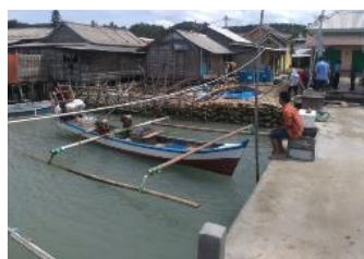
Figure 5. TPI Kramat’s condition.
