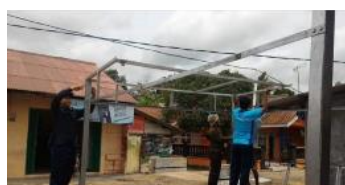
Figure 6. Assembling of solar panel’s frame.
