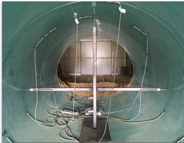
Photo 2. Meters inside the culvert [4].
