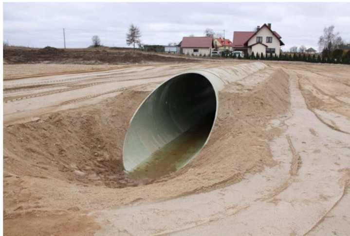
Photo 1. A culvert during construction [4].
