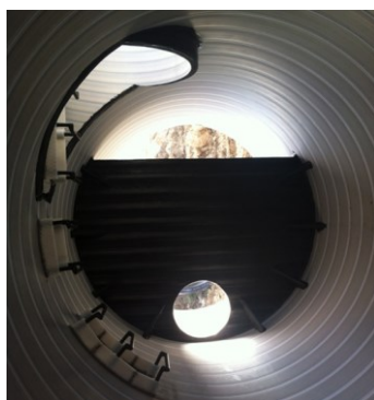
Fig. 2. A piling partition on a sewer with a diameter of 2400 mm.
