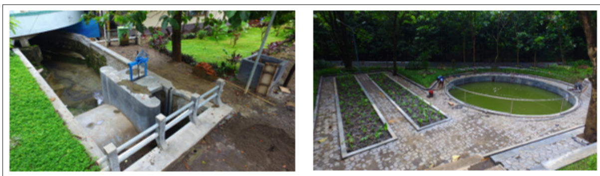
Fig. 3. One of control ponds in Domestic Waste Water Treatment Instalation Universitas Sebelas Maret, Indonesia
