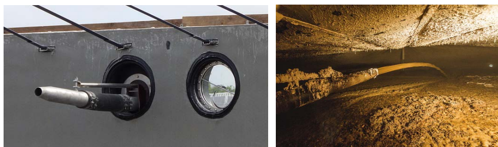
Fig. 2. A sprinkling nozzle (source: http://www.sauter-biogas.de ).
