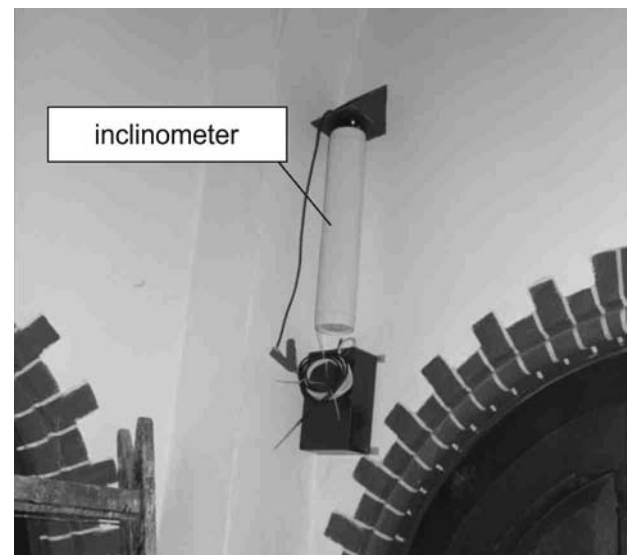
Fig. 3. Installation of inclinometer in quoin of the church tower [4].
