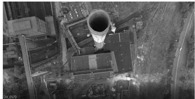
Photo 2. Top of Terma-Dom chimney.
