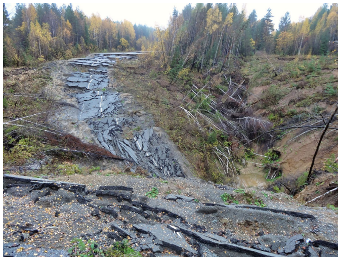
Fig. 4. Formation of the caving zone over the developed deposit in depression zone
