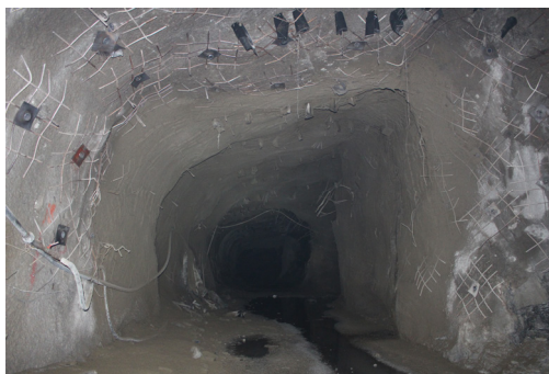
Fig. 4. Improved rock support system of haulage entry of the Yukspor deposit.
