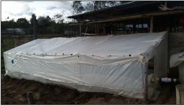
Figure 7. Greenhouse for the bio-digester of Hacienda Terán.
