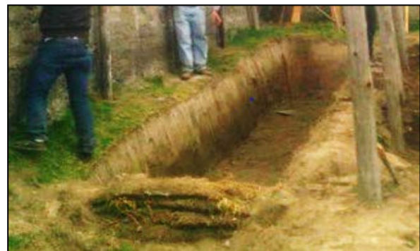
Fig. 6. Construction of the polyethylene digester tank.
