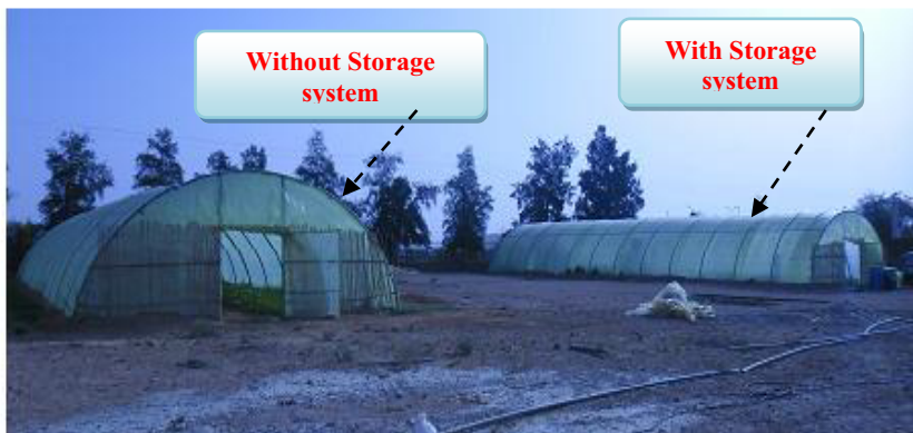
Fig. 5. The two greenhouses test facility in URAER
