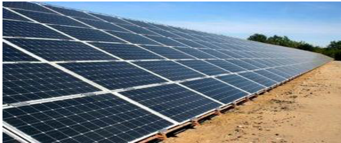
Fig. 3. Solar Power Station in Ghardaia (Algeria).
