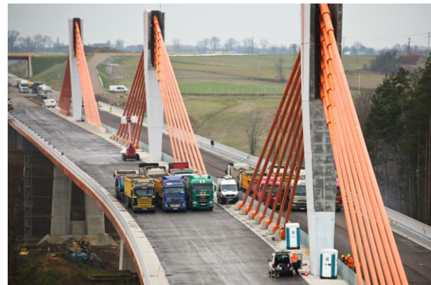
Fig. 4. Full ballast loading during U34 setting.
