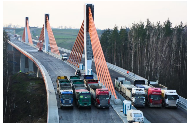
Fig. 5. Full ballast loading during U45 setting.
