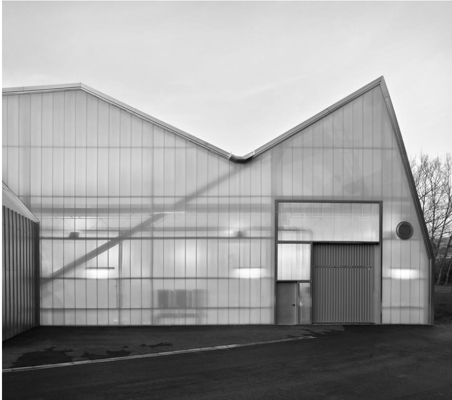
Fig. 2. Wastewater Treatment Plant in San Claudio, phot. By M. Apollonio, 2017 [6]
