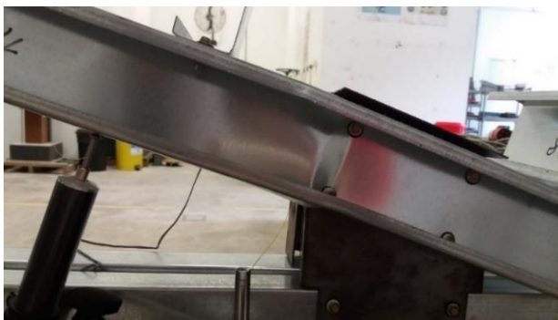
Fig. 9. Local buckling of top chord for heel plate truss specimen.
