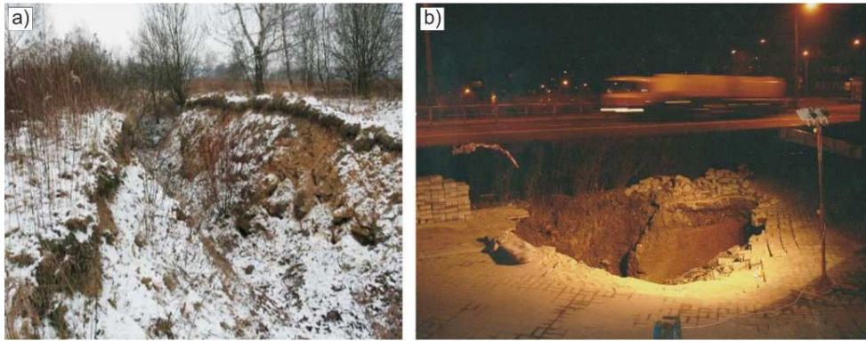
Fig. 1. (a) A ditch on post mining terrain of shallow Zn-Pb exploitation near Bytom town (phot. Z. Pilecki); (b) A cuboid sinkhole over an old shaft near Chorzów town (phot. M. Rotkegel).
