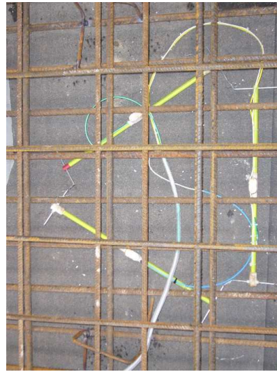
Fig. 4. The rosette installed in the area of the load from the wheels of the left main undercarriage leg.
