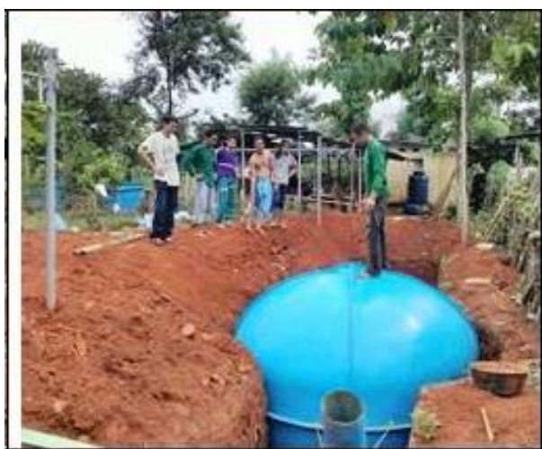
Fig. 3. Biodigester used in the present experiment at local farm in Depok, Indonesia
