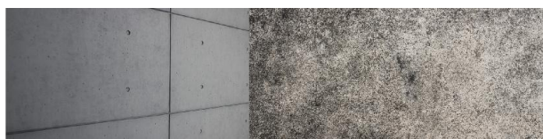
Fig. 4. The retaining walls (left); the texture of outermost concrete (right)
