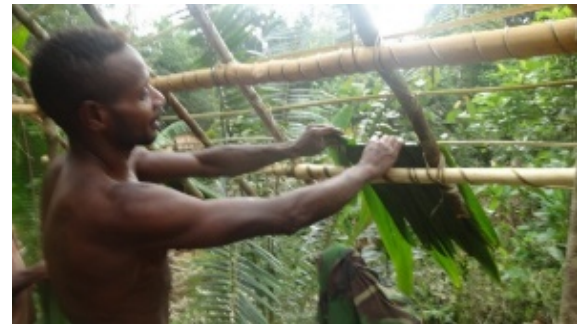
Fig. 7. Roof covering with insert system.
