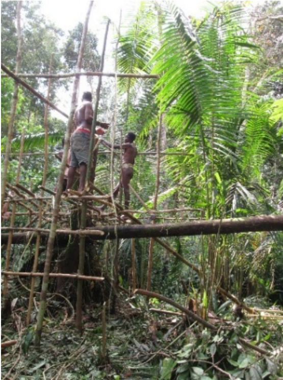
Fig. 5. Floor Structure and additional columns.
