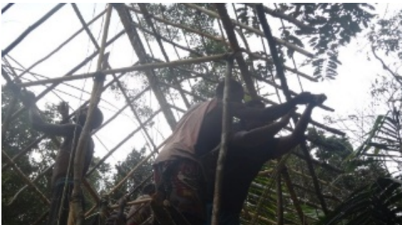
Fig. 6. Make the roof structure
