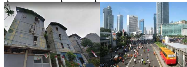
Fig. 2. Physical look of flats Kebon Kacang XI and high rise building on MH. Thamrin Street
