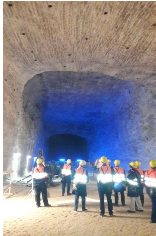
Fig. 3. Room excavation in Kłodawa Salt Mine.
