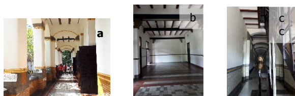
Fig. 4. The Corridor ( a) the room behind the corridor (b) central corridor / The Hall (c)
