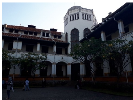
Fig. 1. The A Building of Lawang Sewu
