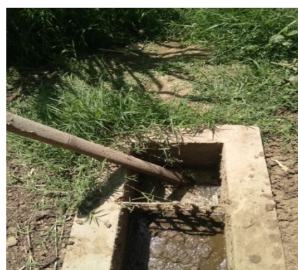
Fig.4. Inlet on Installation
