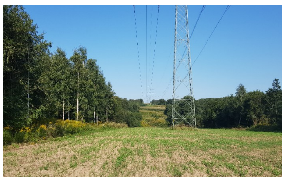
Fig. 4. Reserve along the high voltage line. Source: own study.
