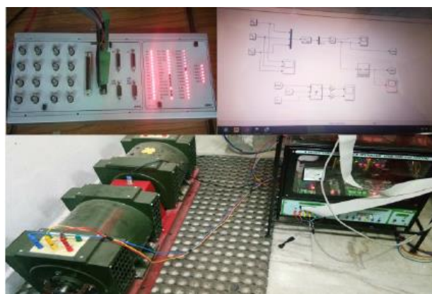
Fig.14. Hardware unit of Three phase Inverter driving IM using DSPACE
