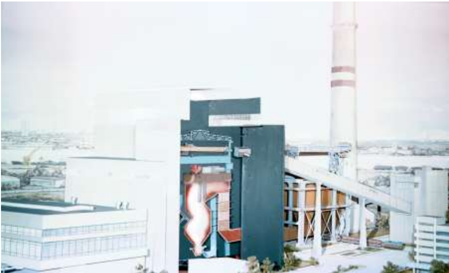
Fig. 2. The layout of the boiler with low-temperature swirl furnace in the boiler room.
