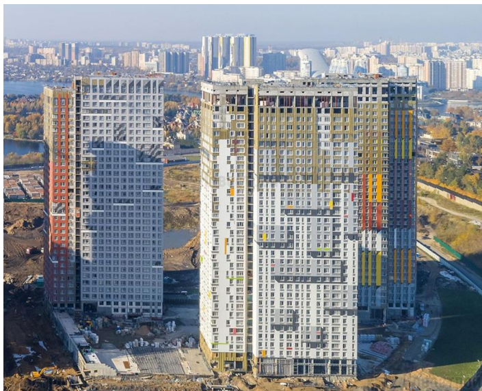
Fig. 2. Apartment complex under construction
