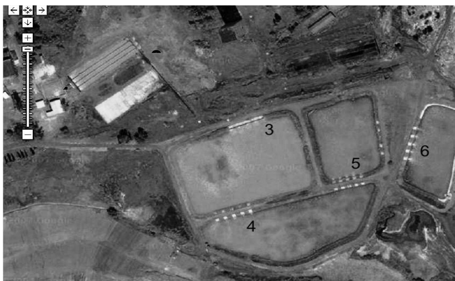
Fig. 1. A complex of treatment facilities on the territory of the former "Glubokaya" mine: 1 - a mixer; 2 - aerator; 3 - the first pond sump; 4 - the second pond sump; 5 - third pond sump; 6 - fourth pond sump
