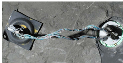
Fig. 6. View of the measuring system installed in the direct roof.
