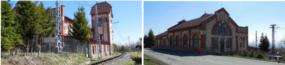
Fig. 2. Traction Substation views from the railway and the road.
