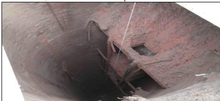
Fig. 3. The inside of the Lubichów III shaft – the entire shaft lining
