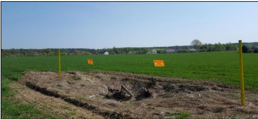
Fig. 6. The sinkhole in the trunk part of the Lubichów IVa shaft.
