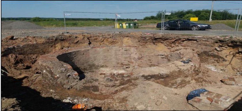
Fig. 4. Exposed Lubichów III shaft barrel.
