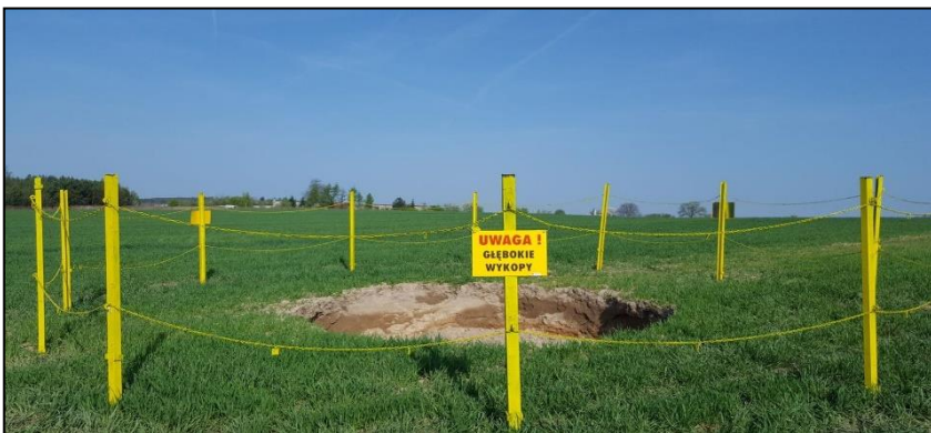
Fig. 9. Secured sinkhole in Lubichów IVa shaft area.
