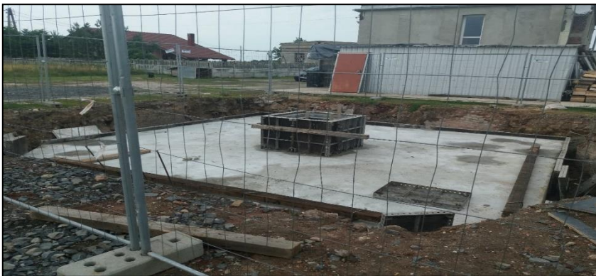
Fig. 5. Reinforced concrete slab with inspection hole securing the Lubichów III shaft barrel.
